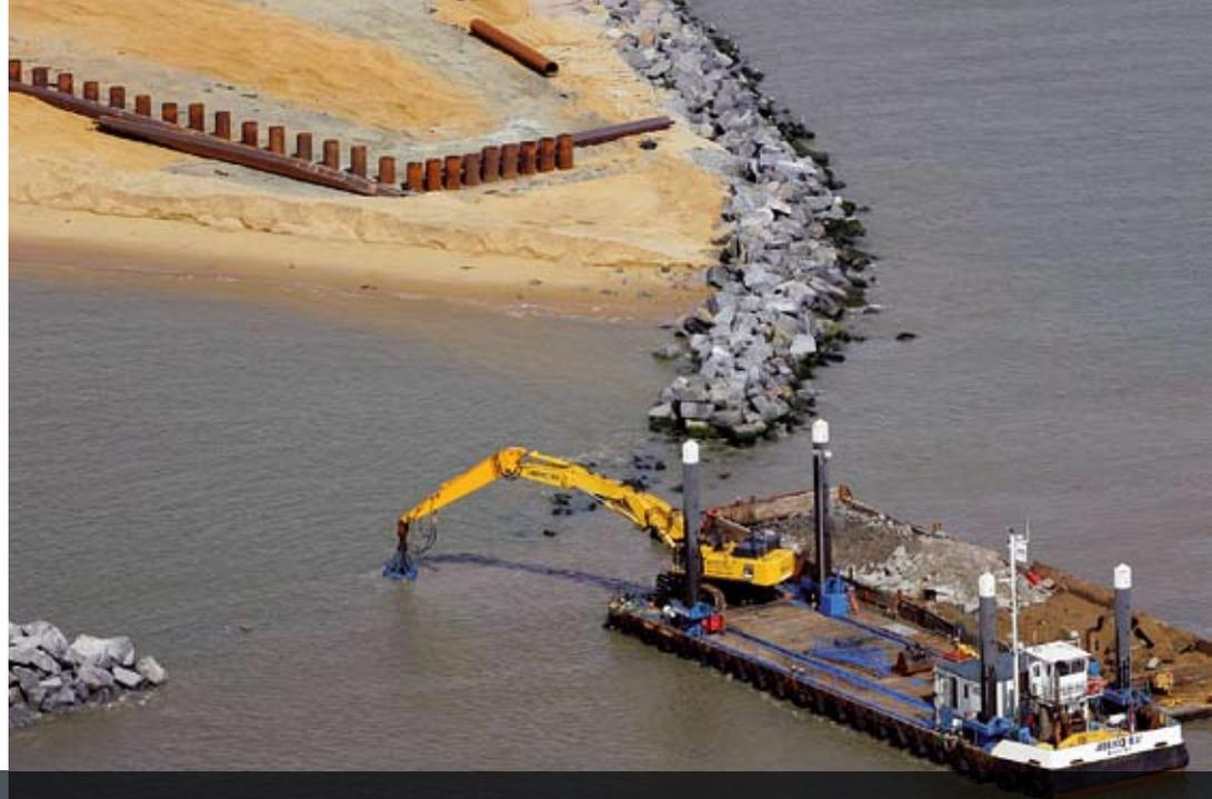
ABEKO SERVER 3 WITH KOMATSU PC800 POSITIONING ROCK ARMOUR OF 6 TO 14 TONNES TO THE BREAKWATER AT THE NEW OUTER HARBOUR AT GREAT YARMOUTH (UK)
