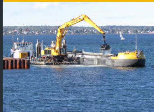
Abeko Server 2, Dredging in Copenhagen (Denmark)
