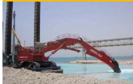
DREDGING IN RAS LAFFAN (QATAR)
