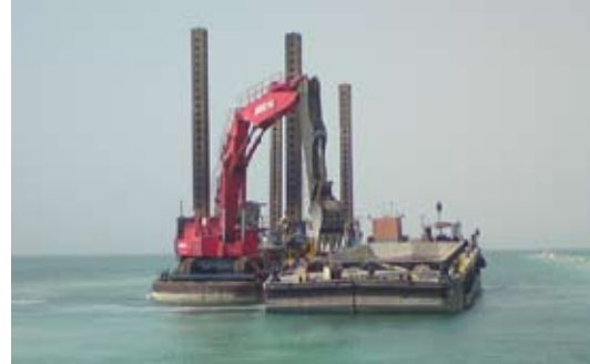
TRENCHING AND BACKFILLING ON THE SAFFANIYAH PROJECT IN SAUDI ARABIA
