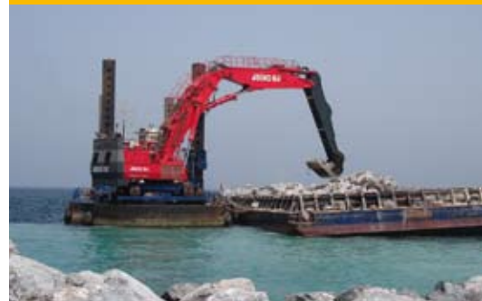
BACKFILLING OF ROCK IN RAS LAFFAN (QATAR)
