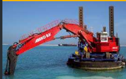
ABEKO SERVER 1, DREDGING THE OUTER HARBOUR IN RAS LAFFAN (QATAR)
