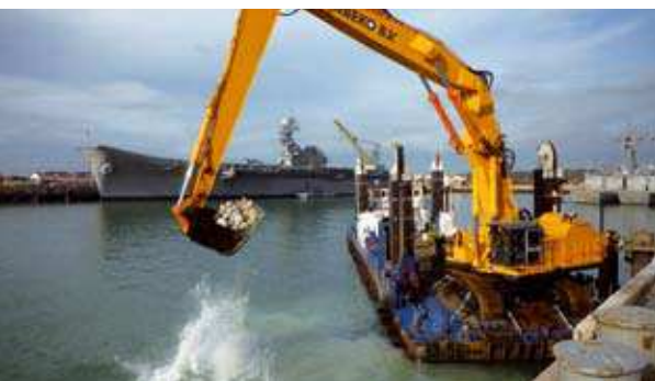
DREDGING ROCK IN ROTA (SPAIN)
