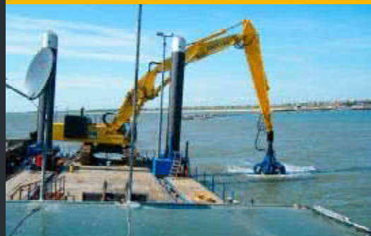
ROCK PLACING IN GREAT YARMOUTH (UK)
